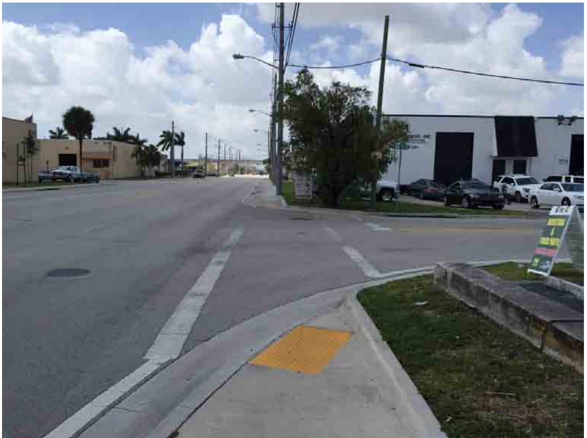
NW 79th Terrace & NW 72nd Ave ADA Improvements: Upgrade DWS, repaint crosswalk
