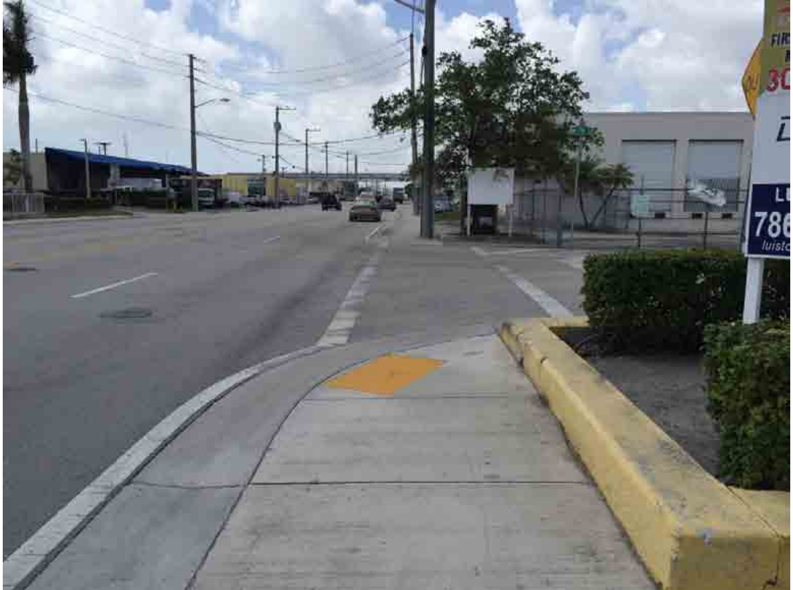
NW 78th Terrace & NW 72nd Ave ADA Improvements: Upgrade DWS, repaint crosswalk
